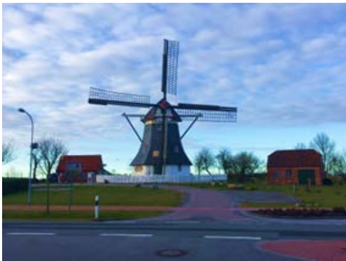
Museumswiese (Backhaus, Mühle, Schmiede)
